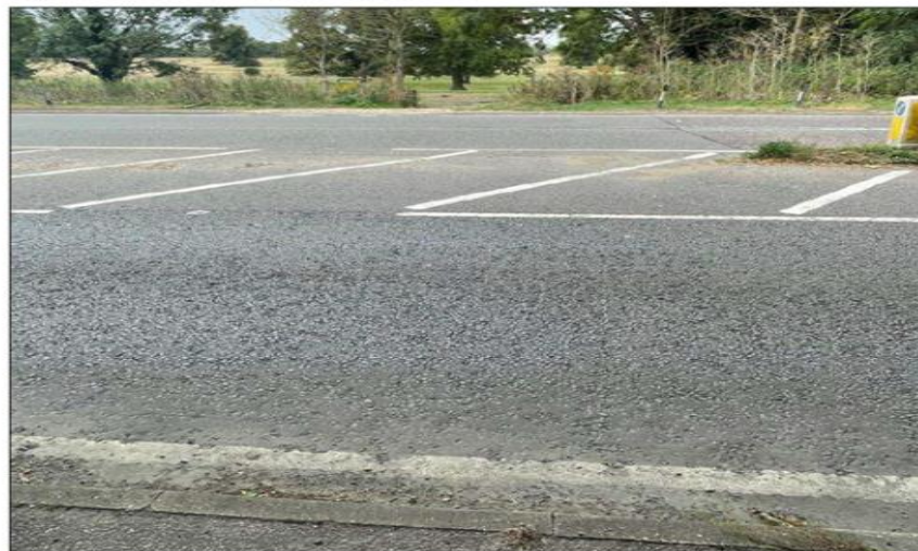
Photo 3.7 – A41 Adjacent to Future Pedestrian/Cycleway Entrance
